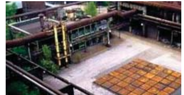
use DUISBERG NORD. Ruhr River Basin sculptural forms indicate use other than original industrial function
