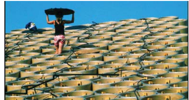
adapt PF1. work architecture. 2008 modular raised food garden in New York City's PS1 gallery courtyard uses sonotube for bed structure
